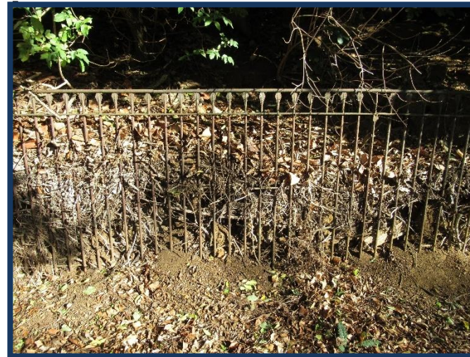
Figure 29: Metal railings along the lane to the church
